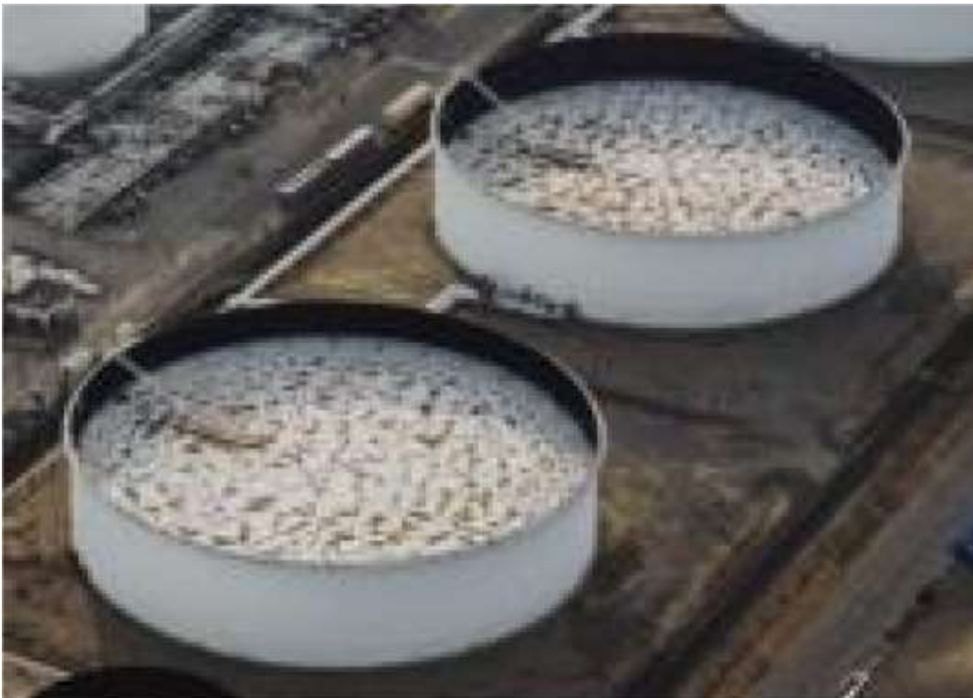
Figure. 3.5: External floating roof tank type.
