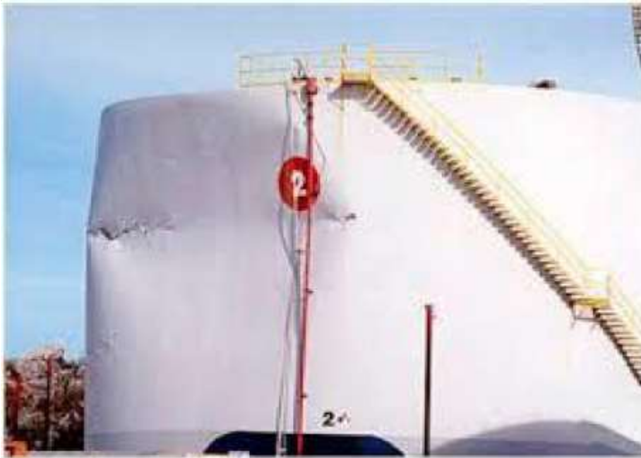
Figure. 3.6: Local buckling of a tank.
