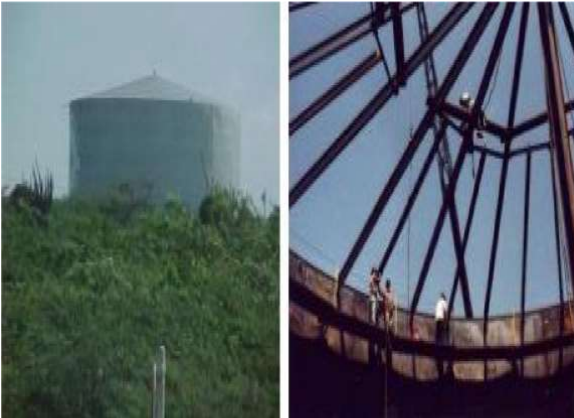
Figure. 3.2.: Fixed roof tank (Cone type).
