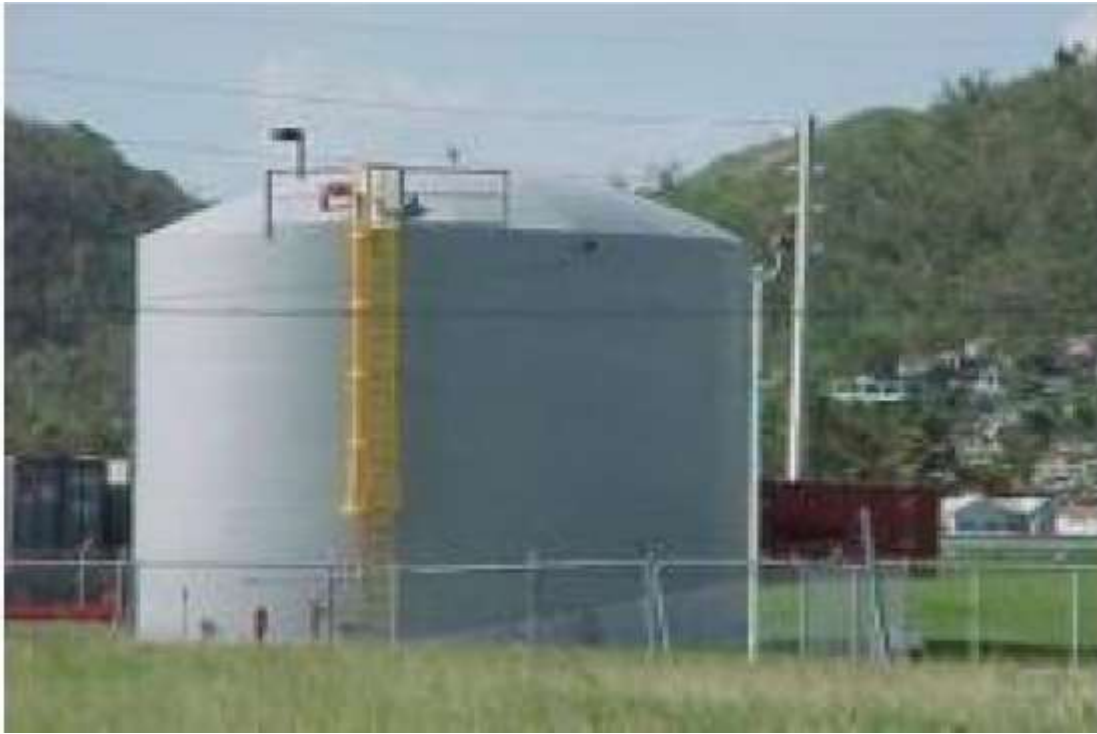
Figure. 3.3: Fixed roof tank (Dome type).
